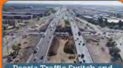
Peoria Traffic Switch and Bridge Demolition
